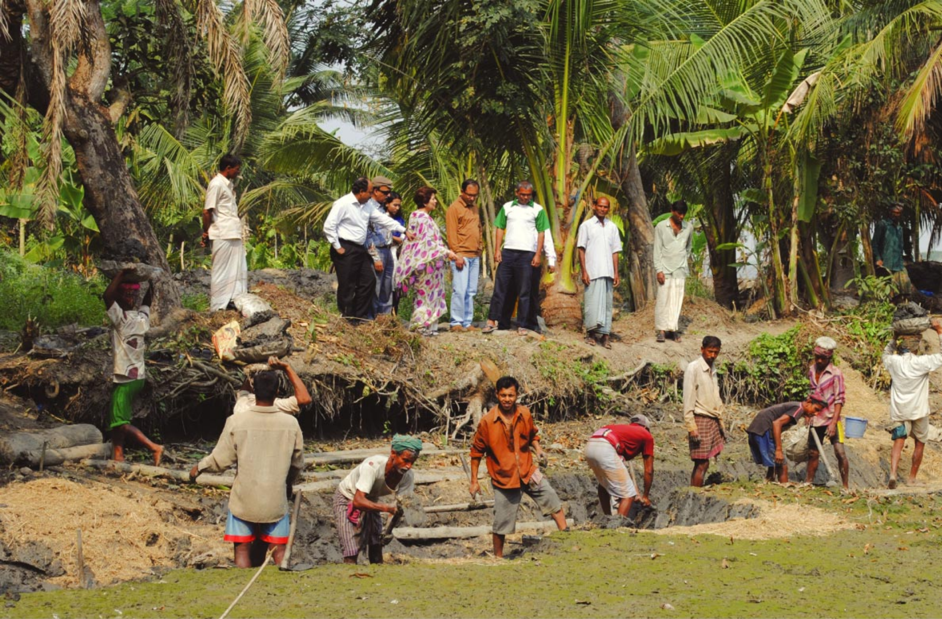
Pond re-exavation at Bon Laudob
