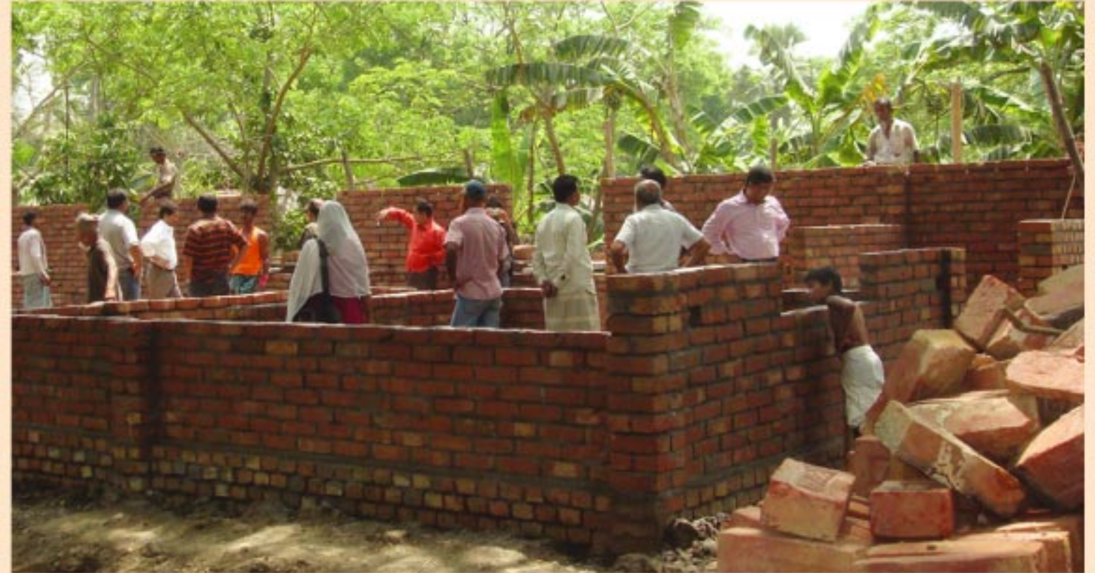
Construction of women's centre at Basatpur in progress
