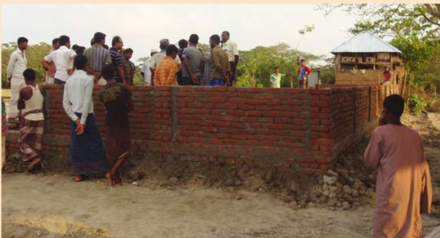
Construction of Sharifpara school building
